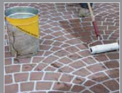
6. Applicazione Resina Sealfloor 100 Sealfloor 100 application
