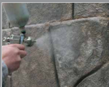
5. Applicazione Hydrofloor Hydrofloor application
