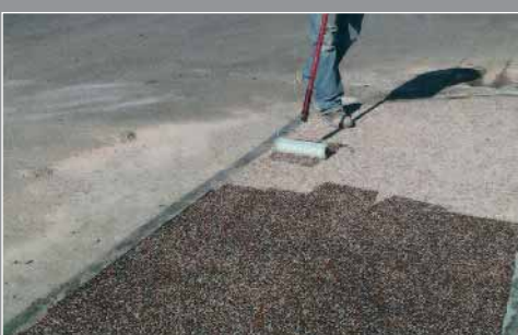
5. Applicazione Sealfloor 100 Sealfloor 100 application
