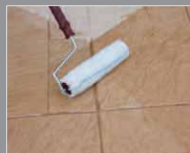
6. Applicazione Resina Sealfloor 100 Sealfloor 100 application
