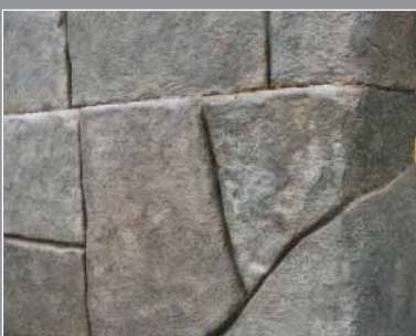
6. Lavoro Finito Finished work
